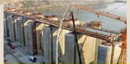
Polavaram project: Andhra Pradesh
